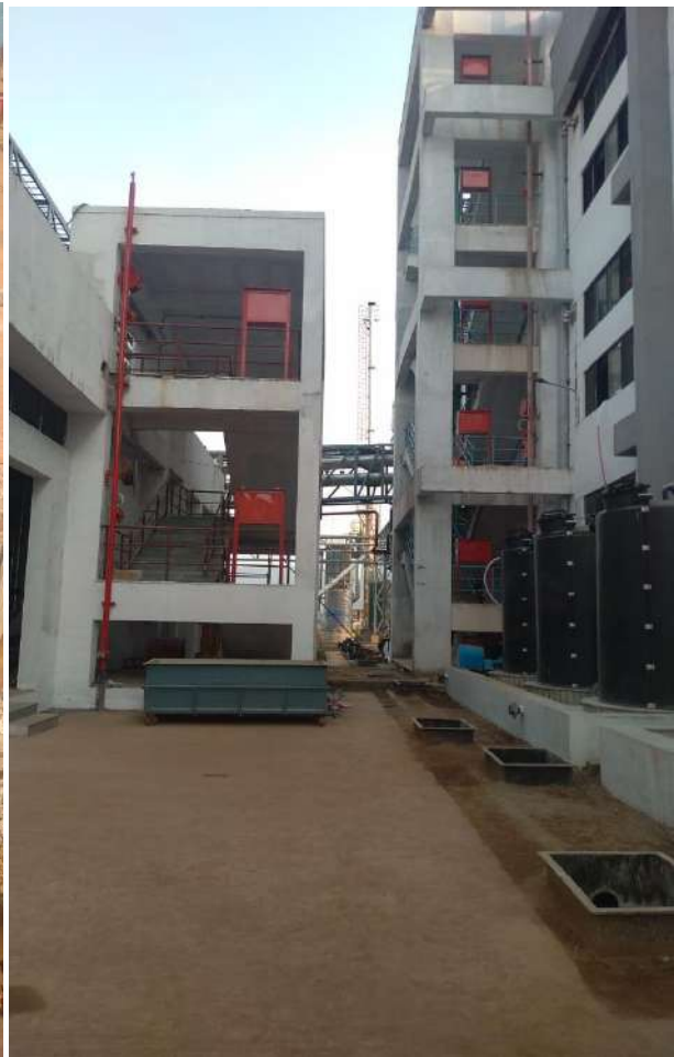
Fire Hydrant box on each floor
