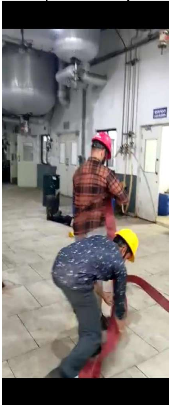
4.First fire hydrant shower on fire spot
